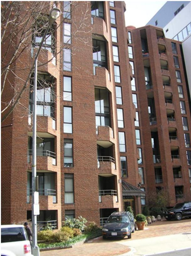
Basic construction is steel and concrete with a brick façade. The roof is a vinyl roofing system with gravel ballast. Glazing is double pane metal framed storefront style in the lobby areas. Tenant spaces incorporate the original structure with double pane metal framed window units. Some tenant units have upgraded window units.
